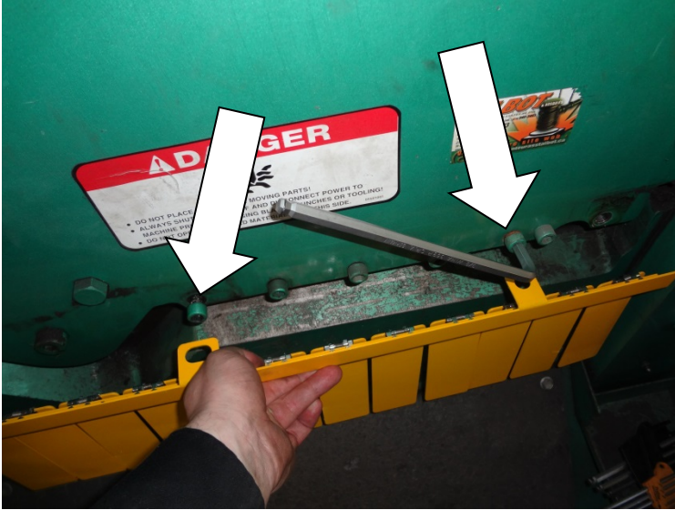
Fig. 9 - Hold up the guard to the machine and determine which two existing bolts to remove for guard installation. Remove the two bolts and install the safety guard using the same bolts. Make sure the bolts are tightened properly.
